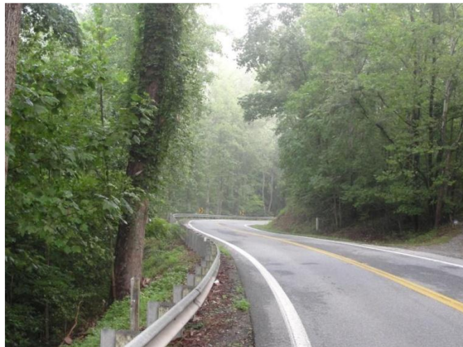
Testing in obstructed areas can lead to noisy GPS data
